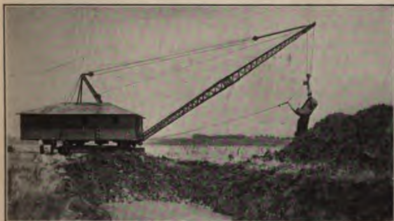
Drag-line Excavator excavating Large Drainage Ditch. Figure 54.
